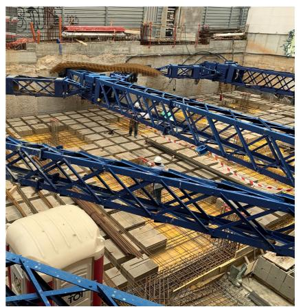
All floors, from the basement to the roof, are executed with a reticular structure and solid slab on roof floors and balconies. The stair slabs and steps are built with concrete poured "in situ".
