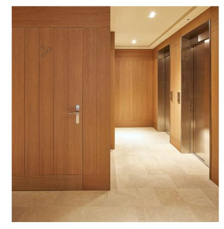
The doors of the apartments, stairs and cupboards are made of oak-veneered fireresistant DM board, following the same design as the rest of the walls.
